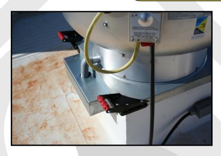
This unique handle plays a vital role in the cleaning, servicing and fire inspection process. It provides a safe way to lift, close and access the inner fan and duct work without damaging the fan bowl and seal, thus helping to prevent future maintenance issues.
