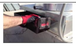
Level box and place second screw. <u>TIP:</u> If you back the screws out a quarter turn it will allow you to remove box off the "keyways" for service
