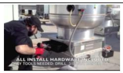
Locate area under drain where rack needs installed. <u>TIP</u>: Install system as high and close to drain as possible to help ensure grease goes into rack.
